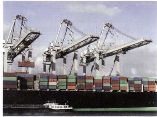
d gantry crane
